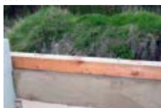
After curing, place the PUR STONE on the concrete base.
