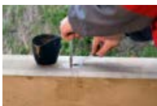
Immediately after application, clean the hole of excess material.
